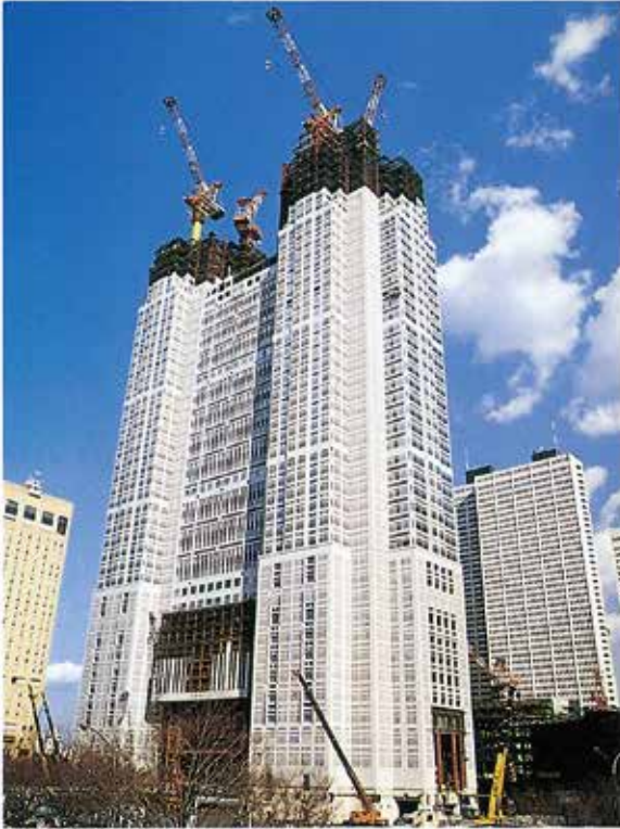
Metropolitan Government Office building
